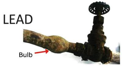
A dull, silver colored pipe that can be easily scratched with a coin or key. Scratching leaves a shiny silver color. Magnets <u>WILL NC</u> stick to lead pipes. Lead pipes are bendable and commonly have a "bulb".
